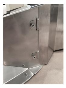
After these three screws are placed in the bales on each side, there is one more screw on the top toward the front on each side that locks in the top panel.
